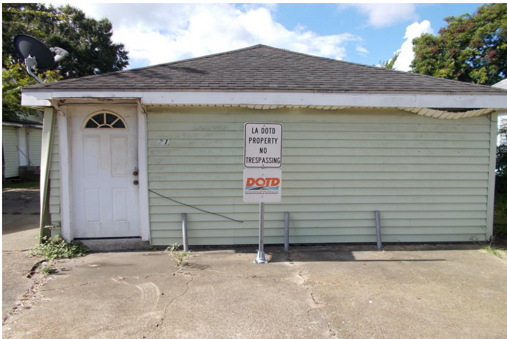
521 NE Evangeline Throughway (Building on slab facing Mudd Avenue)
